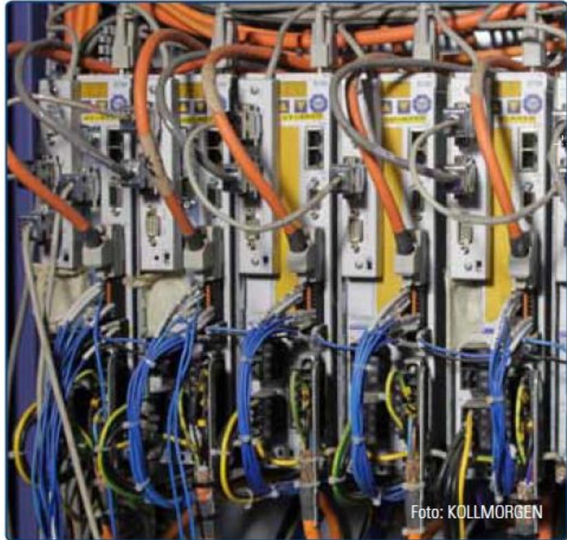
Servodrives S700 are placed with less space in the cabinet way due to their variable, modular design.
